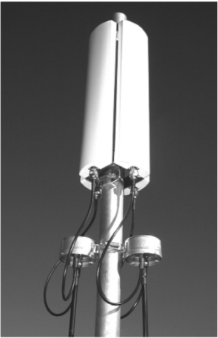
Picture shows four VP470/24 antennas and two two-way power dividers connected for 2x180° coverage.
